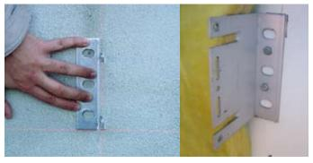
Trace the axis for positioning the vertical profiles, separated by distances depending on the size of the terracotta products and on the width of the vertical joint. Fix the brackets with anchors on both sides of the future position of the profile. Fix the insulation around those brackets.
